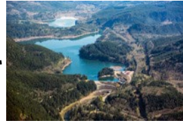
Howard Hanson Dam Green River, Seattle District USACE
