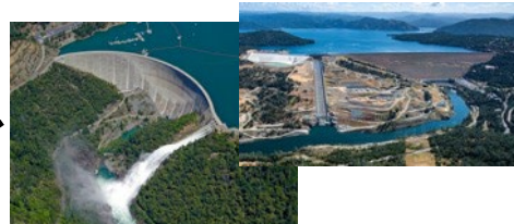
New Bullards Bar Dam Yuba River, Yuba Water Agency Oroville Dam Feather River, CA Dept. of Water Resources Sacramento District, USACE
