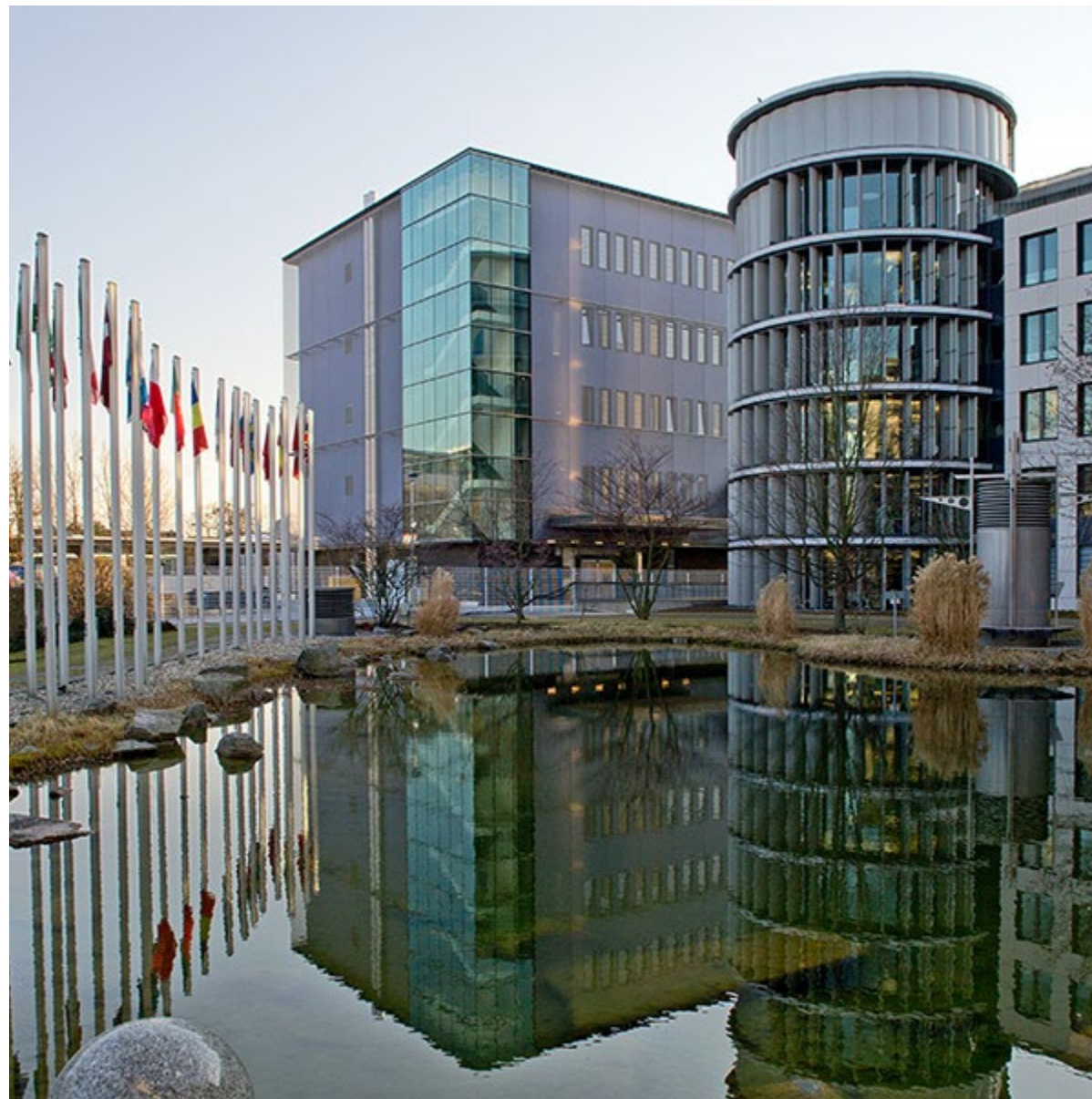
EUMETSAT Data Centre (in the center)
